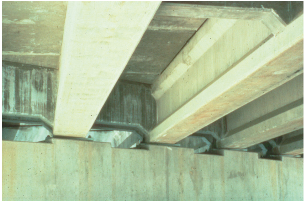
Figure P.1.47 Prestressed Concrete Multi-Girder Bridge
