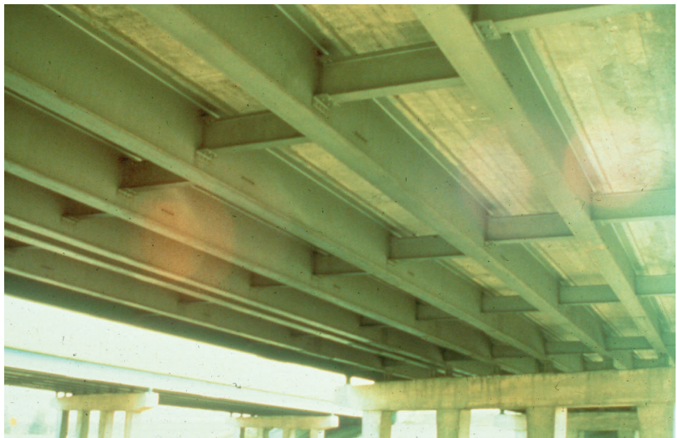
Figure P.1.41 Diaphragms
