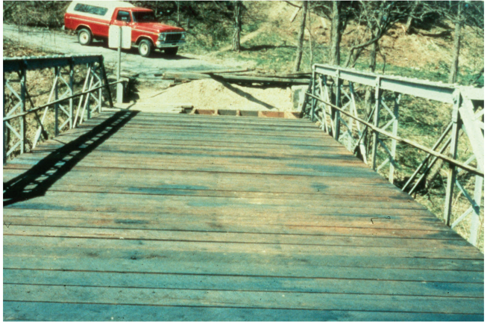
Figure P.1.28 Plank Deck
