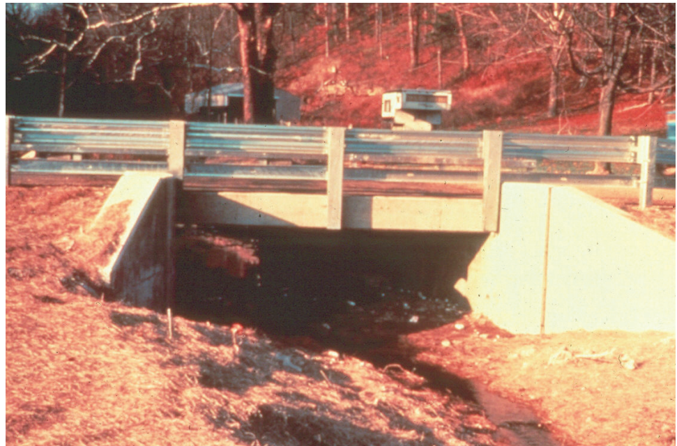
Figure P.1.45 Slab Bridge
