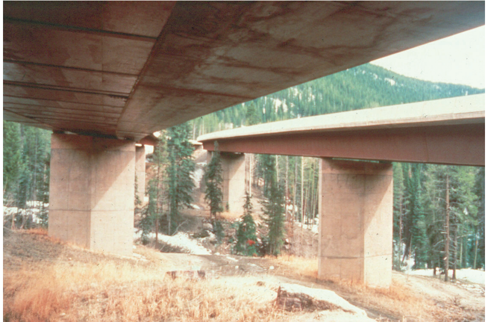
Figure P.1.52 Steel Box Girder Bridge
