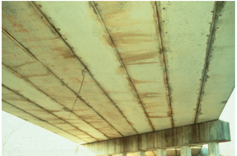
Figure P.1.51 Adjacent Box Beam Bridge
