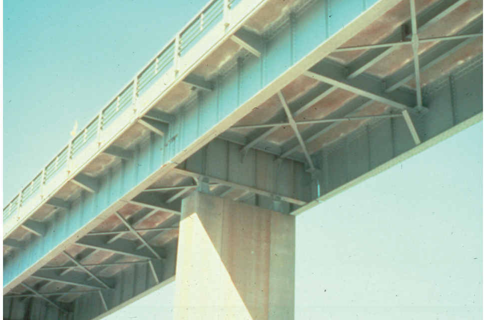
Figure P.1.48 Girder Floorbeam Stringer Bridge
