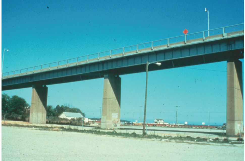
Figure P.1.72 Column Pier
