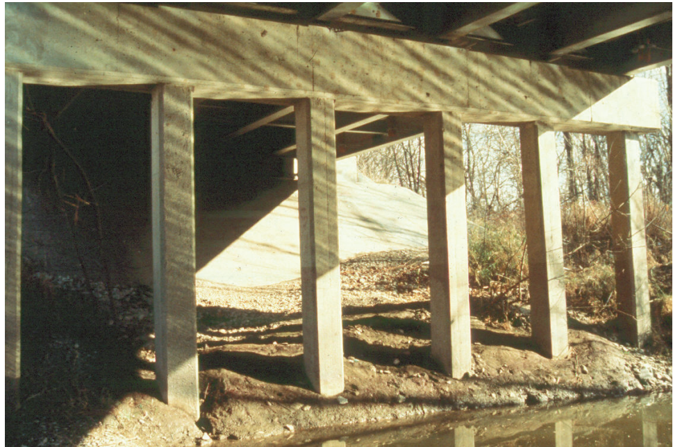
Figure P.1.8 Concrete Pile Bent
