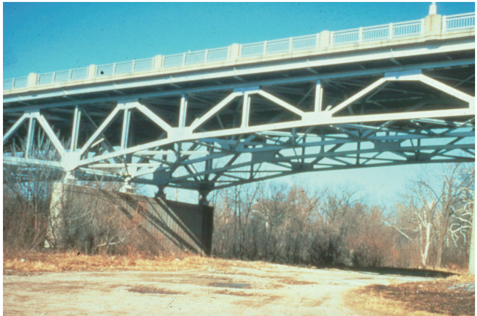
Figure P.1.53 Deck Truss Bridge
