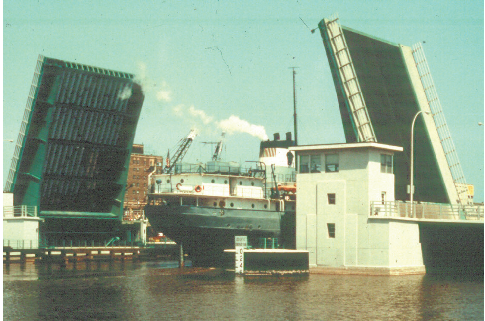
Figure P.1.59 Bascule Bridge
