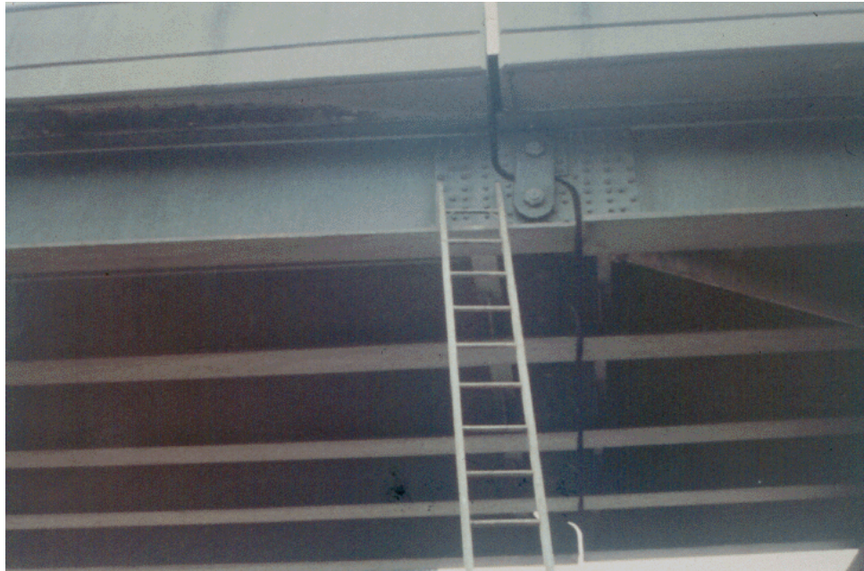
Figure P.1.22 Pin and Hanger Connection
