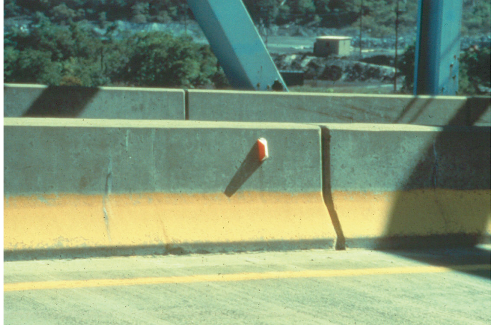
Figure P.1.36 New Jersey Barrier
