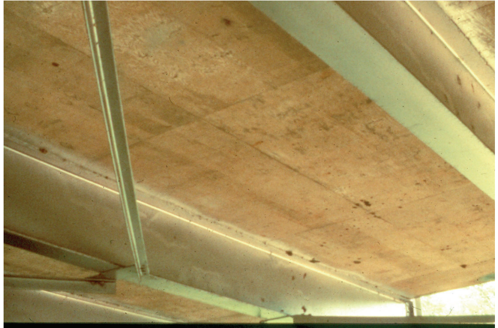
Figure P.1.29 Concrete Deck
