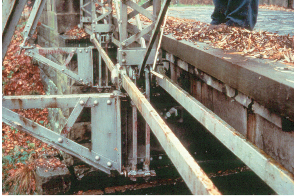
Figure P.1.18 Pin-Connected Truss Members
