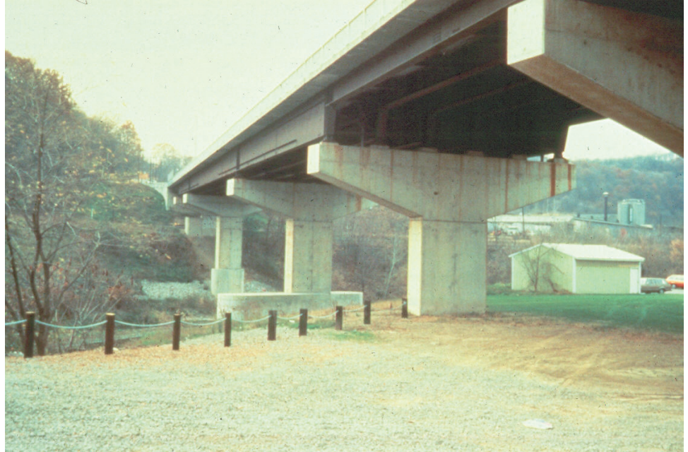
Figure P.1.74 Cantilever or Hammerhead Pier
