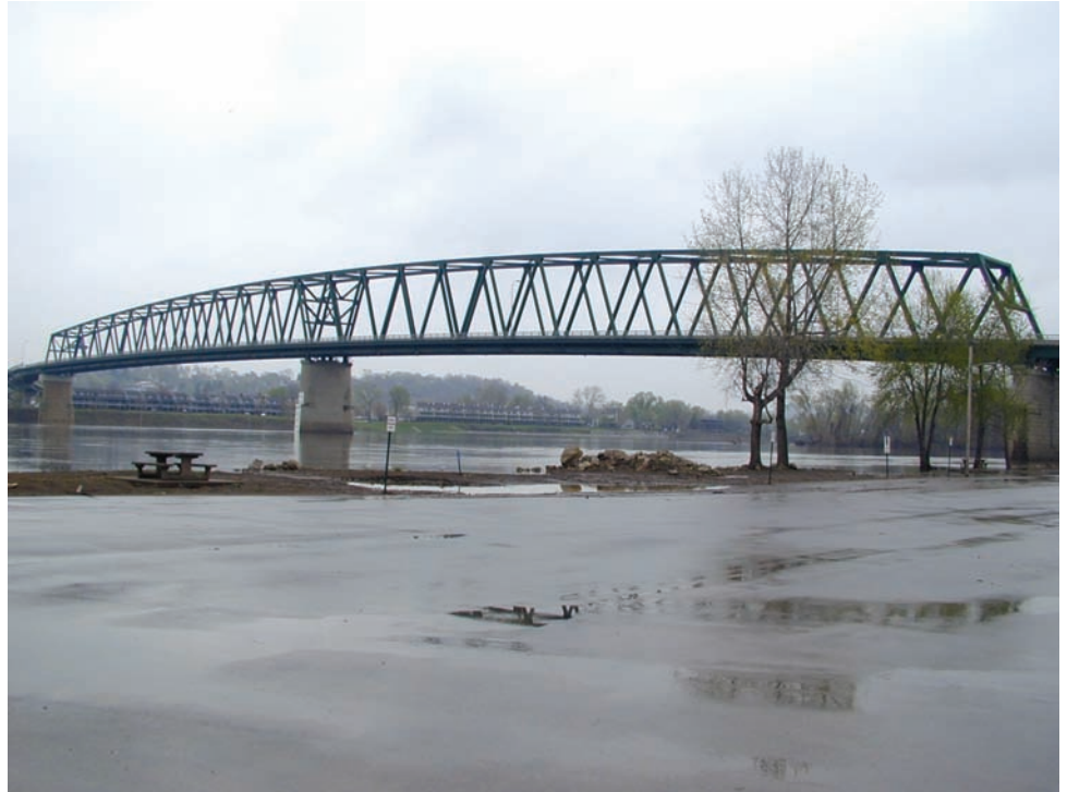
Figure P.1.54 Through Truss Bridge
