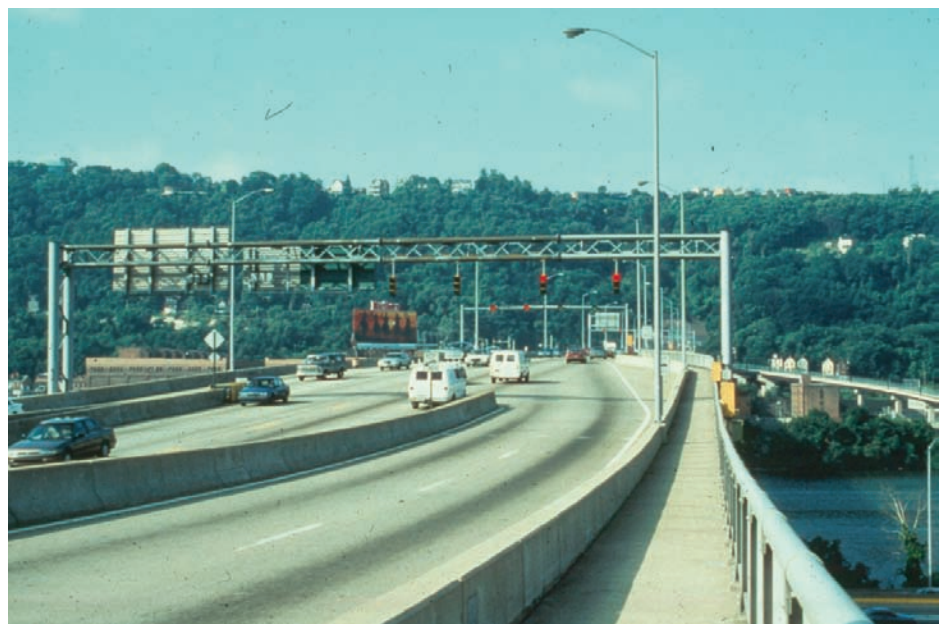
Figure P.1.38 Bridge Lighting
