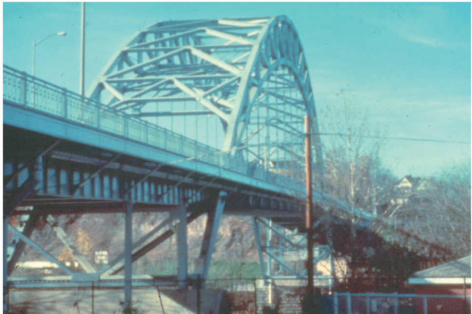
Figure P.1.56 Through Arch Bridge
