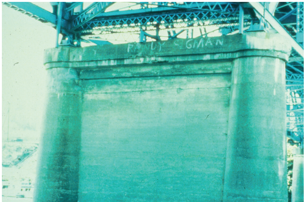
Figure P.1.73 Column Pier with Web Wall
